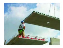
suitable for the majority of new build projects. Requires fixed or mobile crane to lift into position due to weight of manufactured elements as delivered to site.
