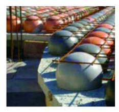
**Type B** – Reinforcement Modules, Comprising pre-fabricated 'bubble-reinforcement' sandwich elements. The modules are placed on traditional site form work, loose joint, shear \* edge reinforcement added and then concreted in 2 stages to the full slab depth. Suitable for suspended ground floor slabs and alteration/refurbishment projects, particularly where site access is extremely restricted. Can be manually lifted into position.
