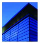
**City Hall and Offices:** BubbleDeck's superior cantilevering ability achieved 3.3 meter cantilevers from a 280mm deep slab with 7.5 meter internal spans between columns. The building provides a City Hall and financial centre for Danske Bake containing 4.000m<sup>2</sup> floor area. The slender slab with out any beams secures maximum light from the facades, which is enhanced by an internal atrium. This project won 'Building of the year 2004 award for offices and commercial buildings.
