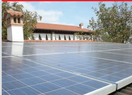
6 kWp plant on pitched roof
