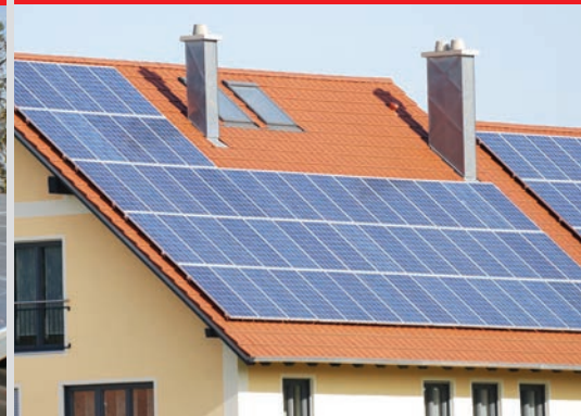
13 kWp plant on pitched roof
