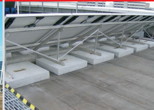
45 kWp plant with STFN
